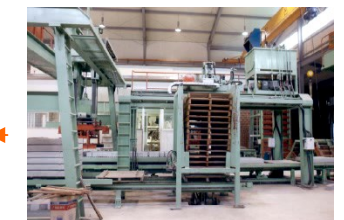
Stock Pallet Magazine holds stock pallets and supplies them one by one to Cuber via Stock Pallet Chain Conveyor
