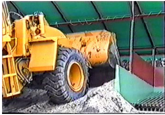
Aggregate supplied to hopper
